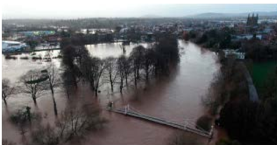
Victoria Bridge and River Wye, Hereford, February 2020 © Will Mears
